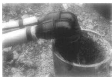
Figure 3. A newly installed polyethene U-tube in a grouted borehole. The two shanks of the tube can be seen, as can the top of a length of steel casing. Subsequently, the borehole would typically be completed below ground level.
